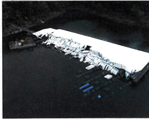
Monroe Lake, Indiana Tornado Damage Salvage
