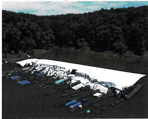
Monroe Lake, Indiana Tornado Damage
