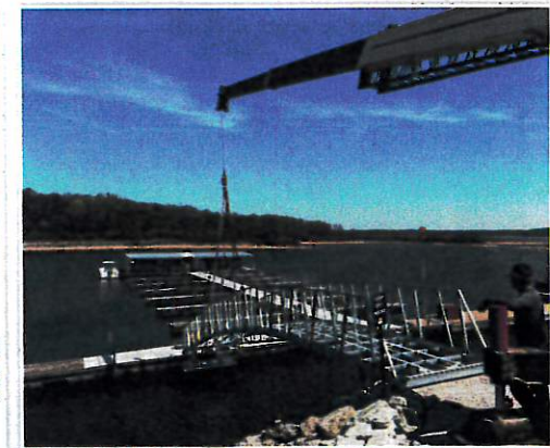
Findlay Marina Bridge Replacement
