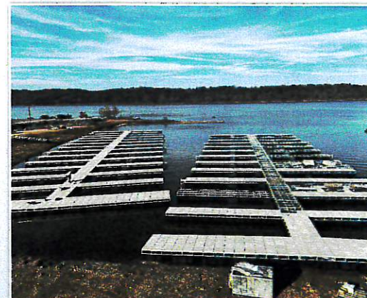
Todd Marina Dock Installation
