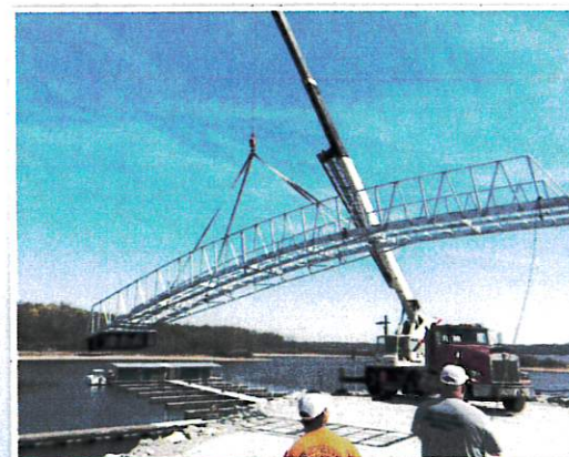
Findlay Marina Bridge Replacement
