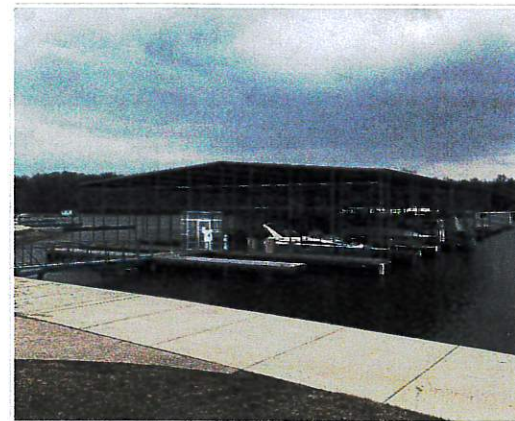
Clinton Marina Dock 4 Replacement, 2014
