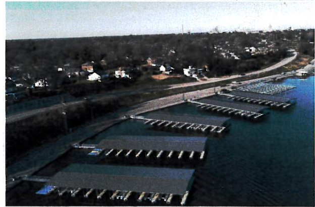
Pier 36 New Construction
