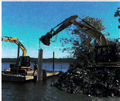
Boat Ramp Replacement
