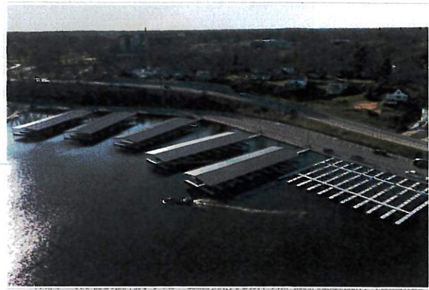
Pier 36 New Construction
