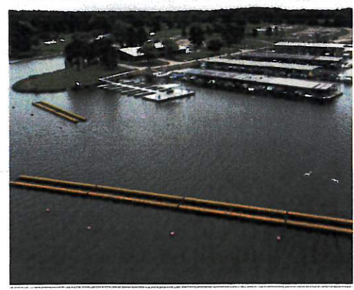
Clinton, Illinois Marina Breakwater
