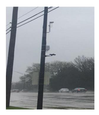
Here are two photographs from the intersection of Hillcrest and Annie Glidden roads. The photograph on the left is the camera on a street light pole. The camera is located in the middle of the pole to capture both lanes of traffic. The photograph on the right shows the transmitter. Again, very easy to spot.
