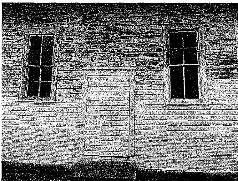
Exterior wall 3-4: Replace glazing on windows with appropriate glazing 25% siding replacement
