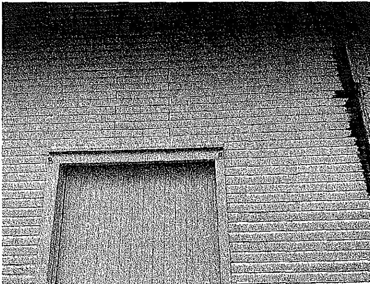
Exterior wall 15-16: Fascia replacement 12 rafter tails 25% siding replacement Corner trim post 15
