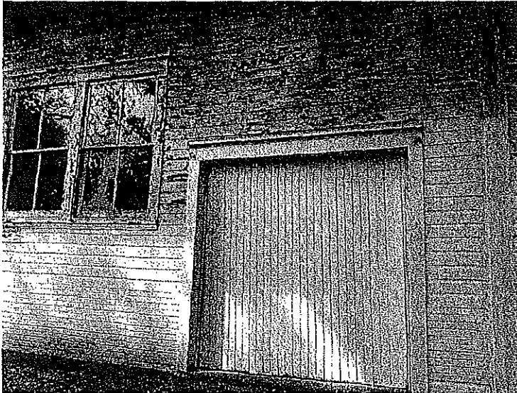
Exterior wall 6-7: 2 pcs rafter tails Fascia replacement 25% siding replacement Corner trim post 7 Hip rafter tail post 7
