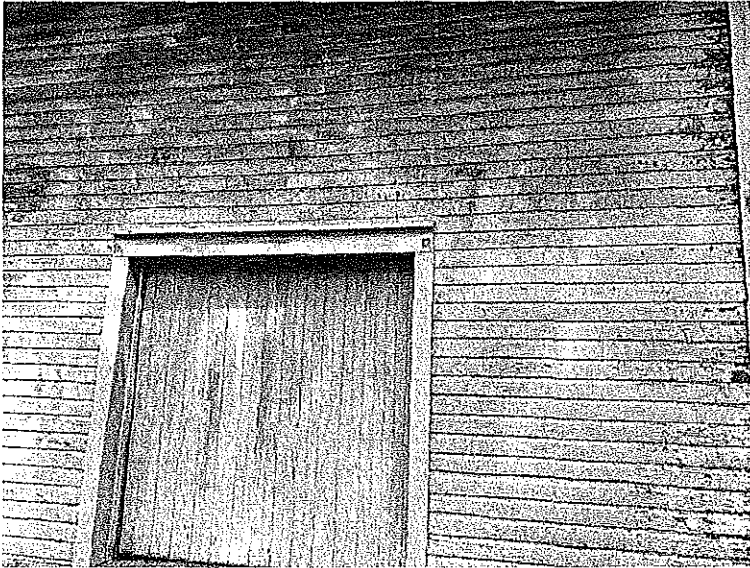
Exterior wall 12-13: 25% siding replacement 12 rafter tail replacement
