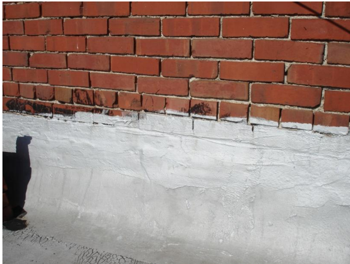
21. Detail view of membrane flashing at 2 nd story wall.
