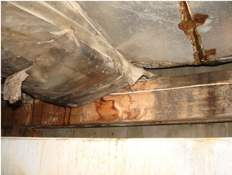
6. Broken beam apparently bearing on and deforming header above overhead door.
