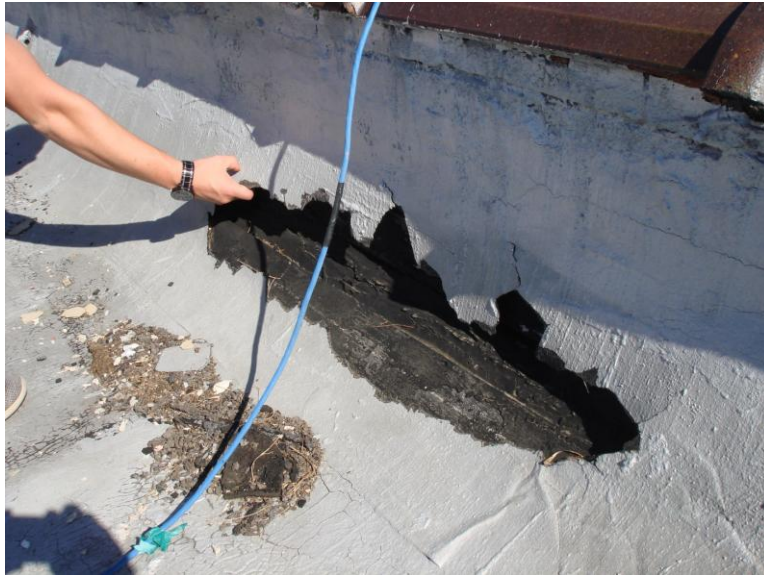
17. Membrane flashing pulled away from parapet, brittle, and broken.
