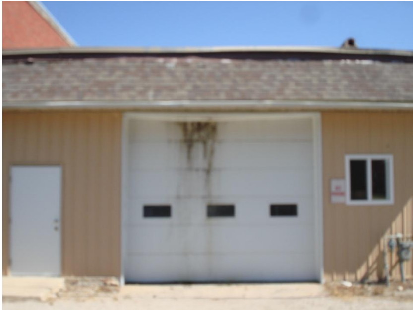
11. Roof eave distorted by collapse of beam and roof deck.
