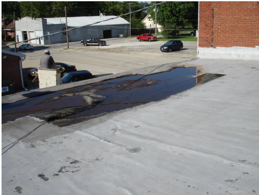
12. Depression in roof above broken beam filled with water.
