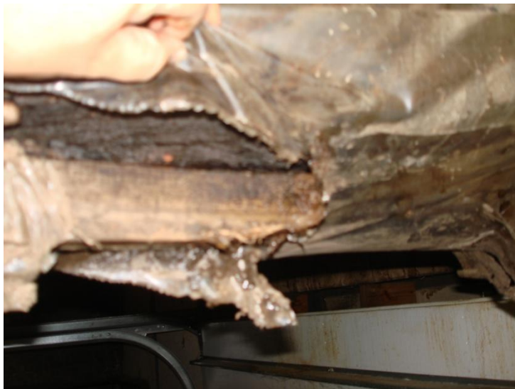
8. Plastic sheeting torn away to reveal break in beam and release trapped water.
