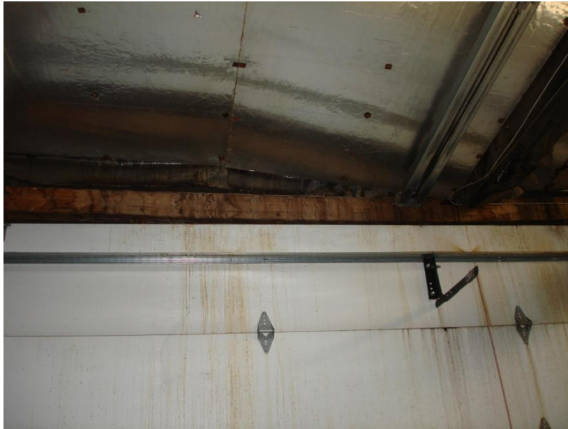
3. Detail view of collapsed ceiling above overhead door.
