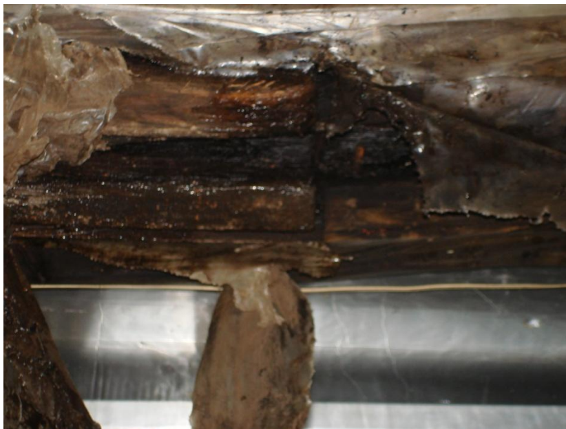
10. Rotted wood and corroded fasteners revealed at break in beam.
