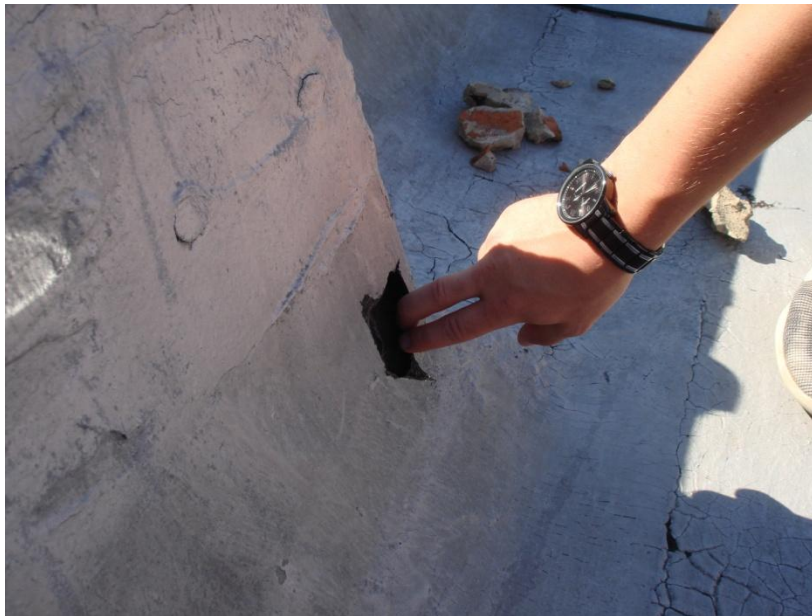
16. Membrane flashing, pulled away from parapet, has become brittle. Breaks in the flashing are large enough for small animals to enter.
