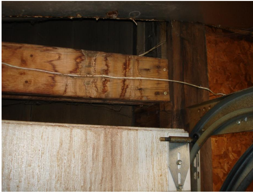
7. Fasteners at west end of header above overhead door pulling out of jamb framing.
