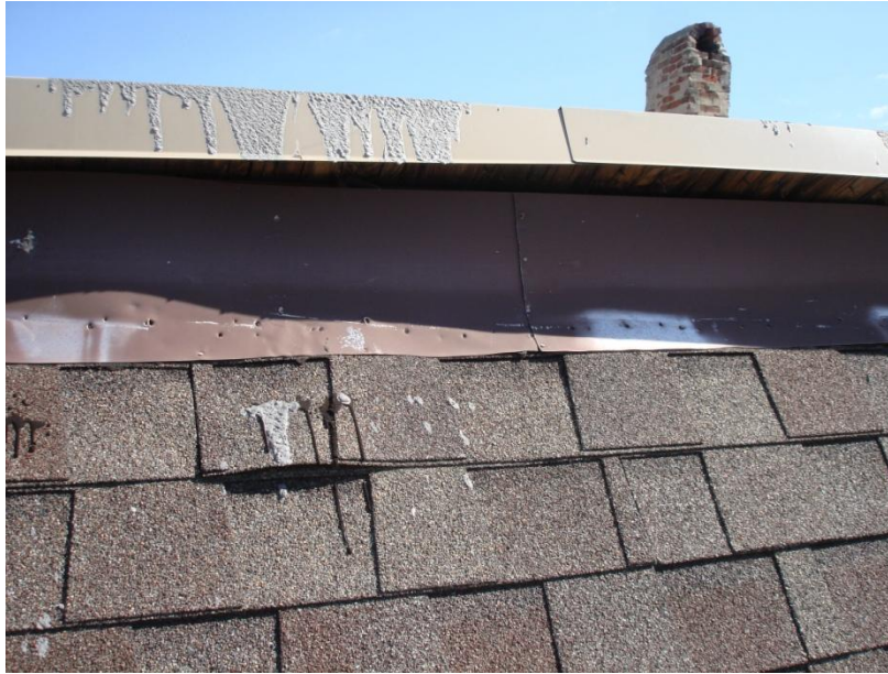
15. Roof eave distorted by collapsed beam and decking now drains up-hill.
