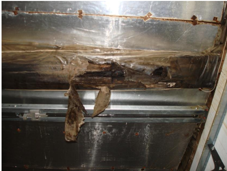
9. Plastic sheeting torn away at break in beam.
