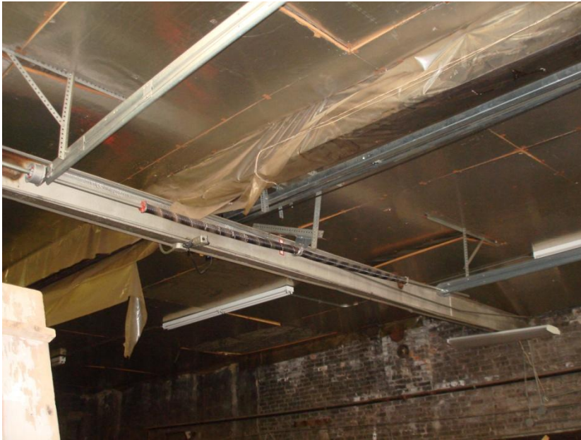
5. Beam supported by steel frame.
